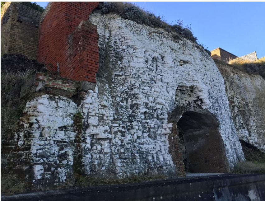
To one of the Tower Bungalows. Blocked.
