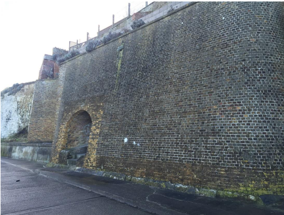
Blocked. Where the newer flats (Winston Court, Spencer Rd) are.
